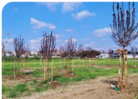
1. Aprilia, Italy, in progress: the Construction Company, to increase the value of building land, created an arboreal infrastructure before the construction of the buildings.
